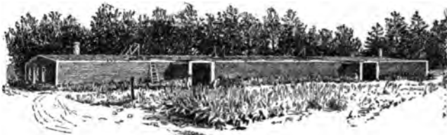
2404. A half-cellar storage.
